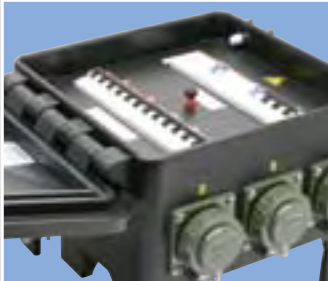
Fuse protection beneath hinged-on cover
