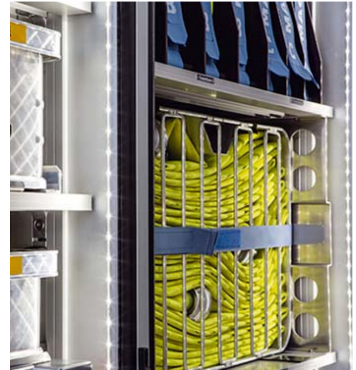
/ LED light strips give the equipment lockers anti-glare illumination and ensure safe working conditions, both day and night.
